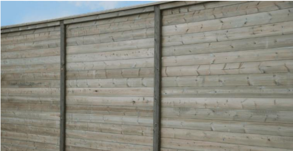
Figure 4 -Close boarded fencing (northern boundary).
