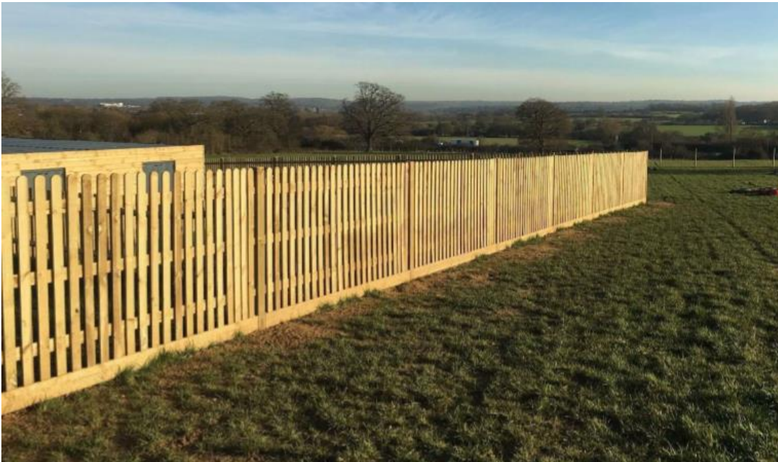
Figure 2 - Palisade fencing (Oxshott site).
